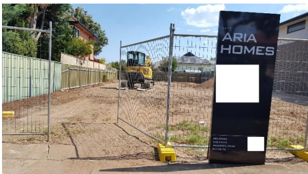
‘La Maison Invisible’, with an idle trenching machine
