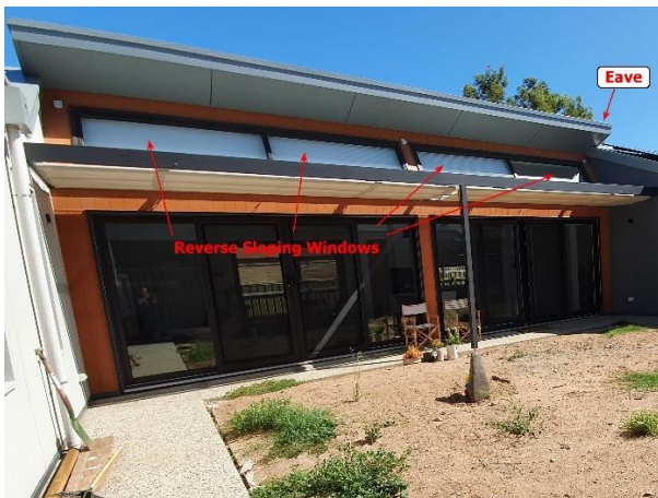
The upward sloping eave
